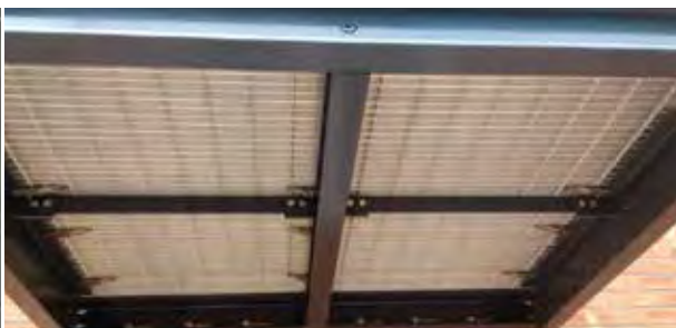
Balcony decking is quick and easy to install with Neaco fixing clips or directly onto steelwork or pedestals.
